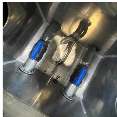
Inside Pod Centre Access Hatch
