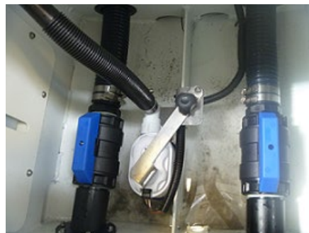
Inside Pod Centre Access Hatch
