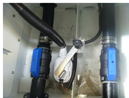
Inside Pod Centre Access Hatch
