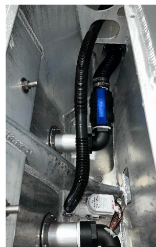
Inside Pod Centre Access Hatch
